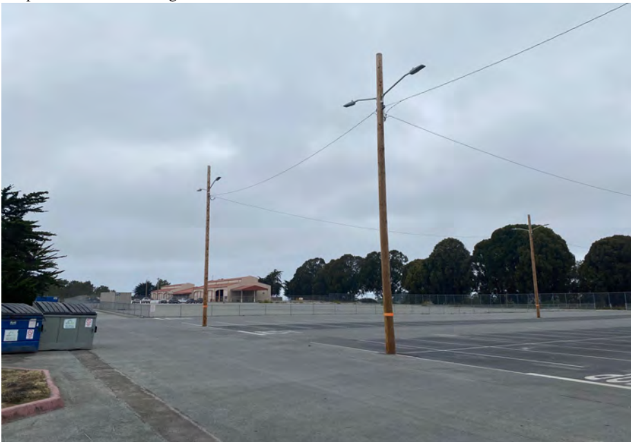
View of existing parking lot and City Public Works Corporation Yard looking west from the Promontory.
