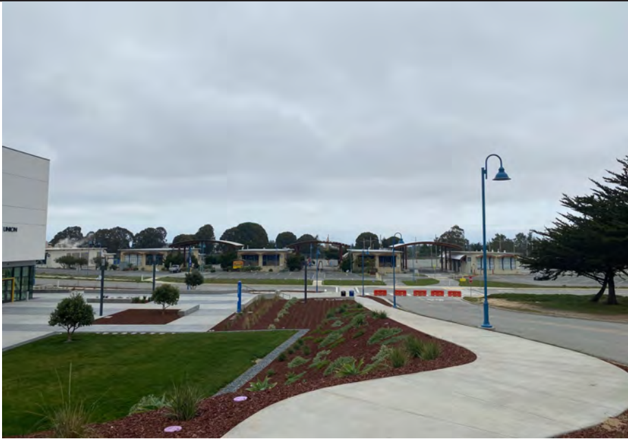
View of site from the Otter Student Union looking north with existing Visual and Public Art Center in background.
